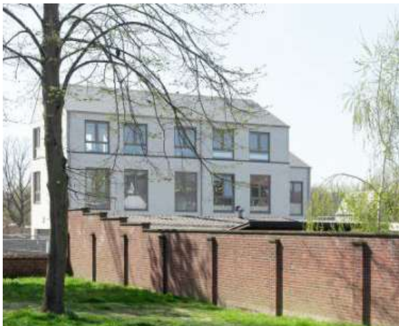
Spoortuin Puurs, Plusoffice architects
